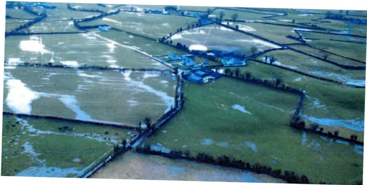
Coolpowra (west of site)
